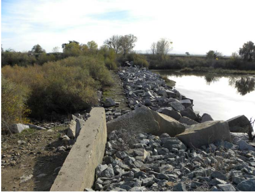
Figure 2-7. Paradise Cut Weir Looking North (Photo taken December 3, 2012)
