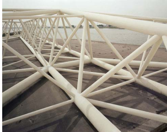
Figure 4: Maeslantkering protects Rotterdam from storm surge (Sayler, 2006)
