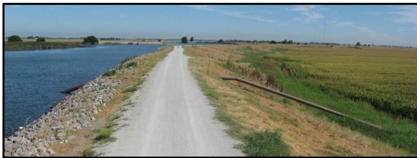
Figure 2. Subsidence on Staten Island, depicting a diversion siphon.
