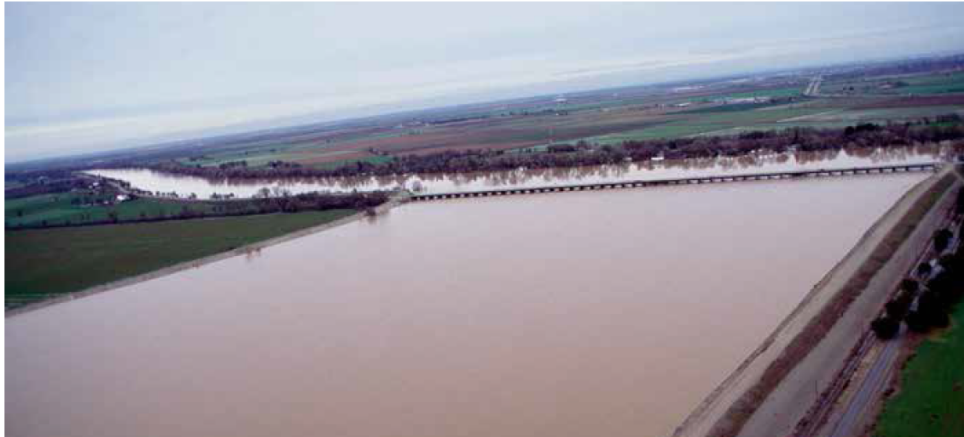
Figure 2.14 Bypass operating during flood of 1997 (DWR)
