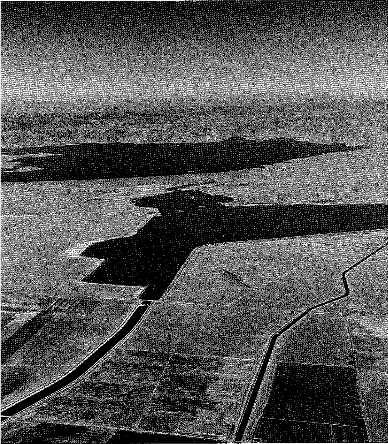
San Luis Dam and the O'Neill Forebay are part of both the Central Valley Project and the State Water Project. San Luis Reservoir stores water diverted from the Delta during the winter when irrigation demand is low. Water is then released later in the year to serve water contractors in the Central Valley and southern California. In addition to the reservoir, a portion of the California Aqueduct known as the San Luis Canal is jointly operated to serve both the Central Valley Project's San Luis service area and the State Water Project customers further south. (DWR photo)
