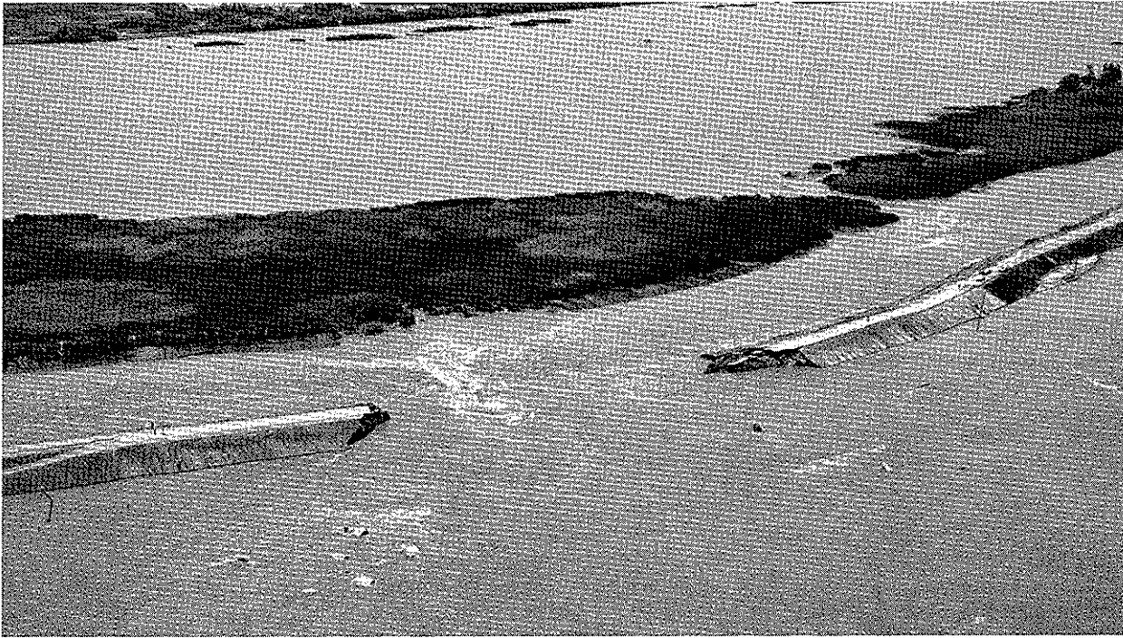
Levee break at Andrus Island in the summer of 1972. The collapse of the levee on the San Joaquin River flooded Andrus and Brannan islands and pulled salt water into the Delta. Upstream reservoir releases pushed the salinity back in the Sacramento River but the only way to remove salt water trapped in the San Joaquin Delta was to pump it into the export canals and send it southward. (DWR photo)
