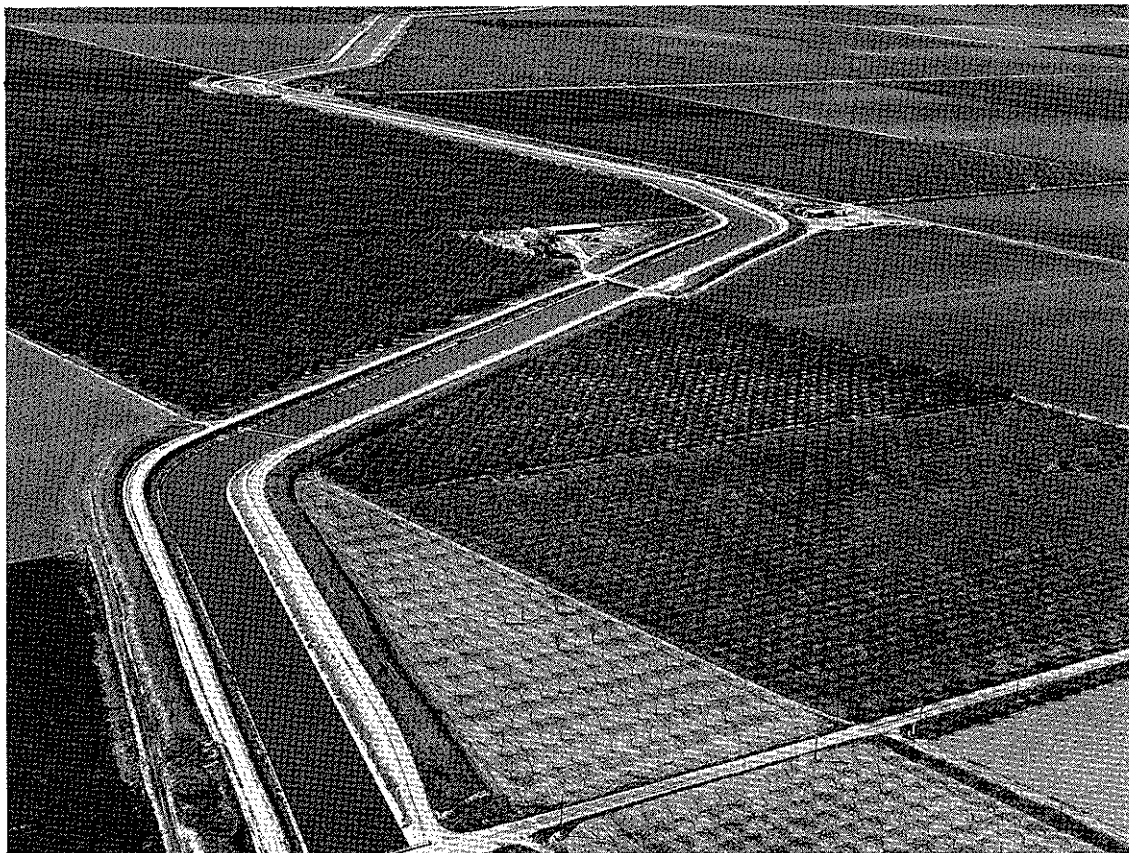
Delta-Mendota Canal, Central Valley Project. From the Tracy Pumping Plant, the canal runs 117 miles to the Mendota Pool on the San Joaquin River west of Fresno. It provides water for the San Joaquin River to replace flows impounded by Friant Dam, as well as serving irrigators along the west side of the San Joaquin Valley. (USBR photo)
